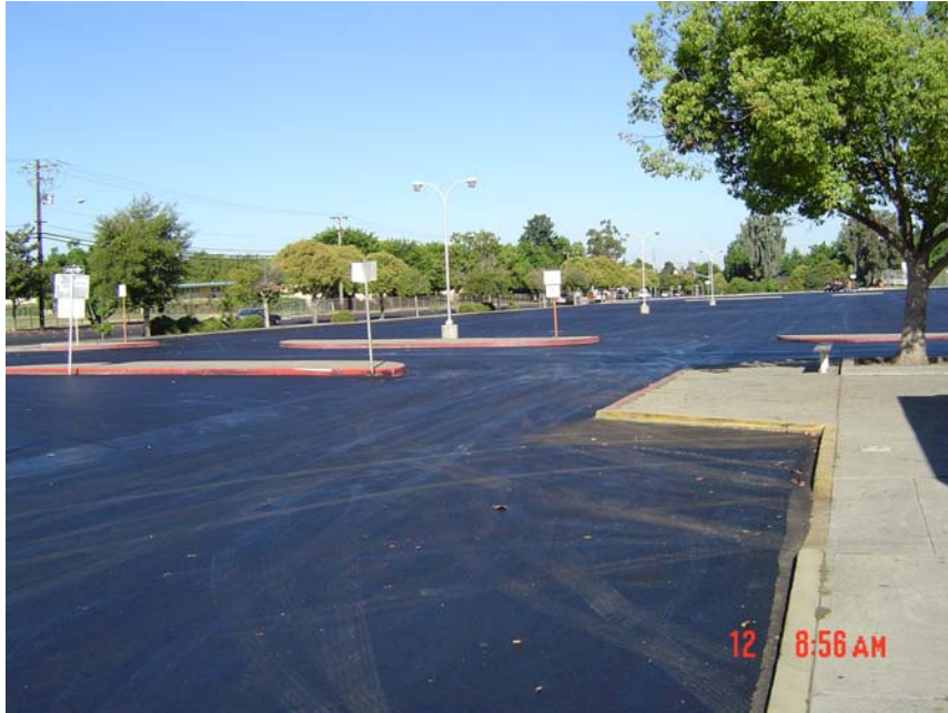
New Parking Lot
