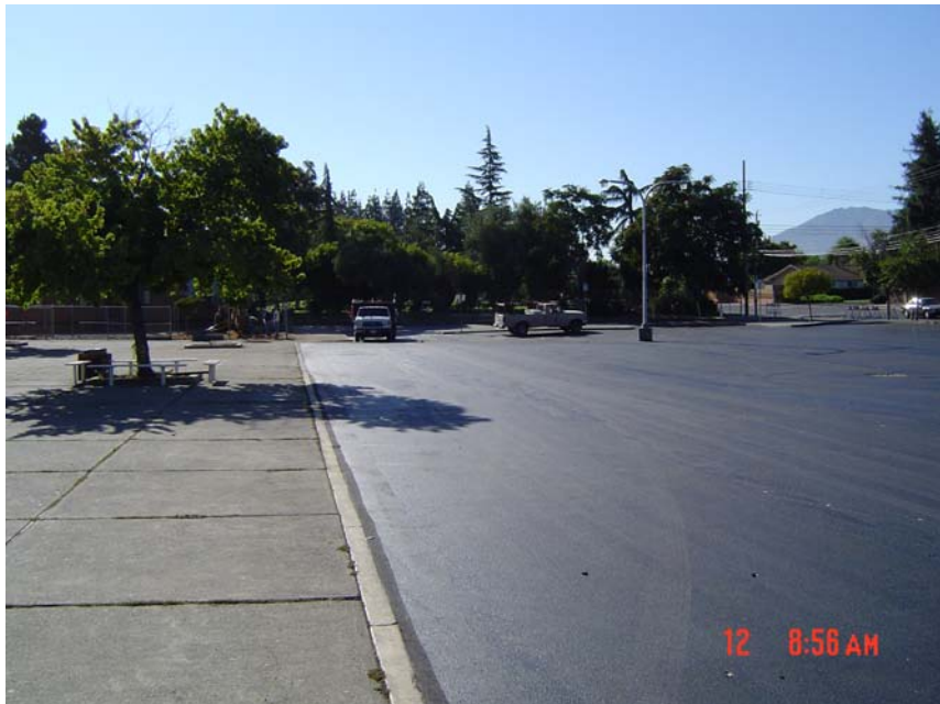
New Parking Lot
