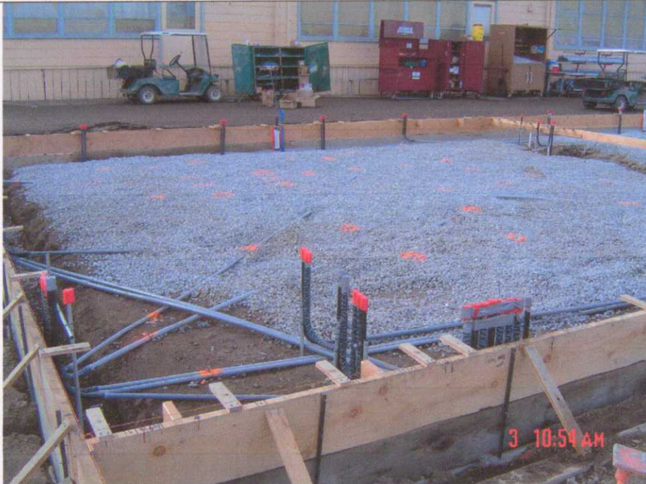
Formwork for Prototypical Building foundation slab
