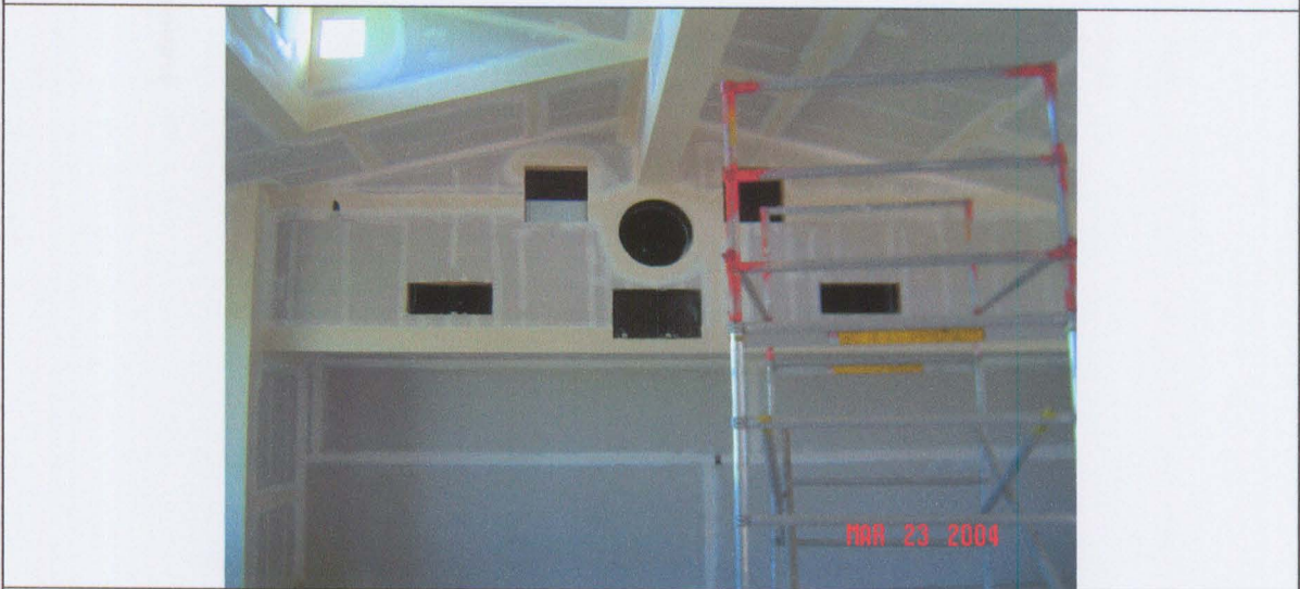
Interior of a prototypical classroom being taped and prepped for painting.
